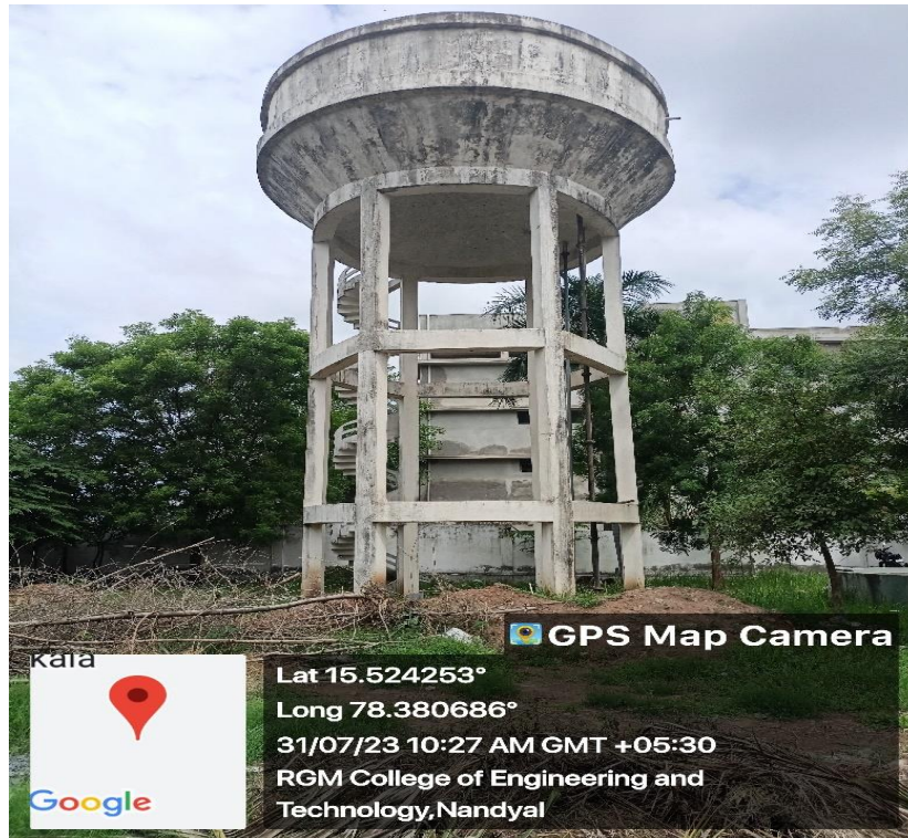
Overhead Tank in front of CE Block
