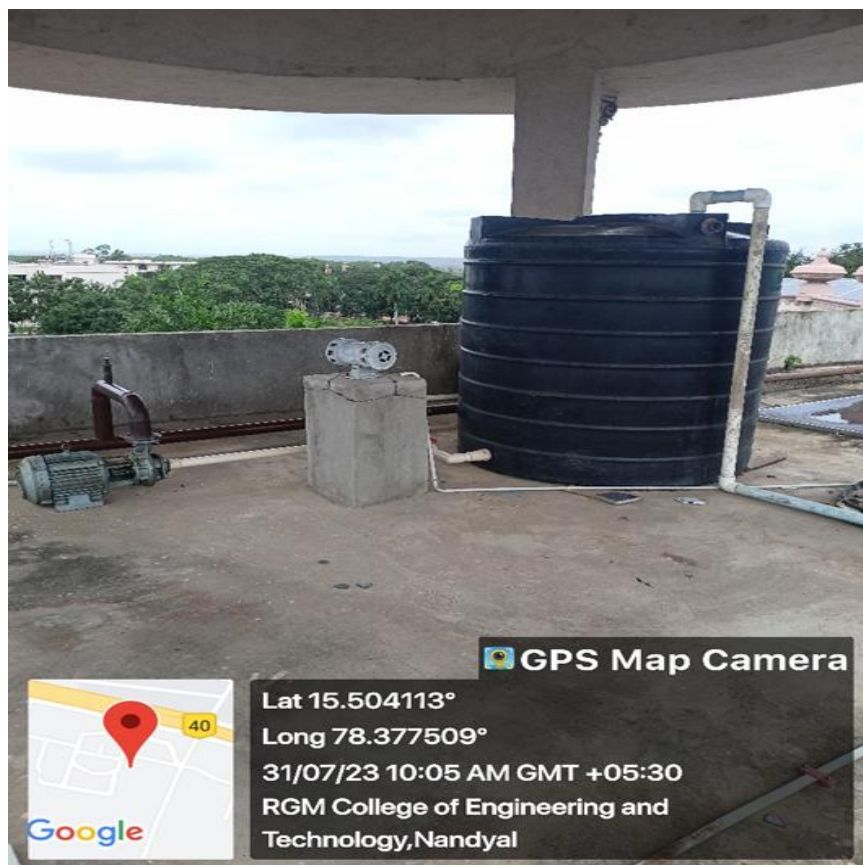
Water Tank on top of RB Block
