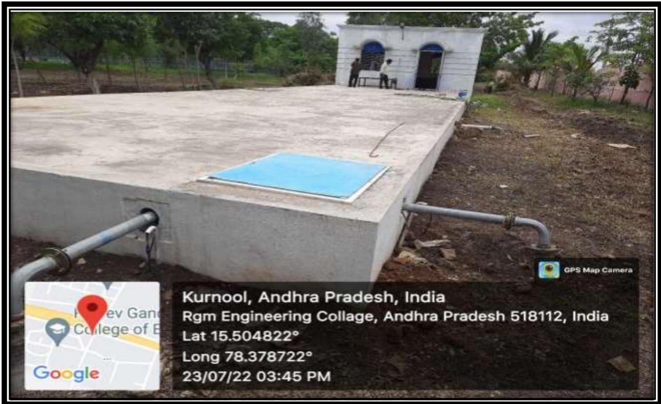
Sump at the Back side of the Canteen
