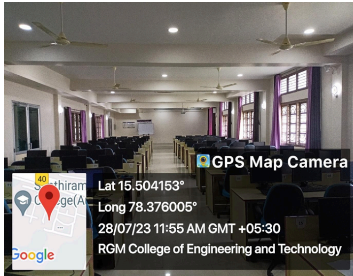
LED Bulbs in the Laboratories
