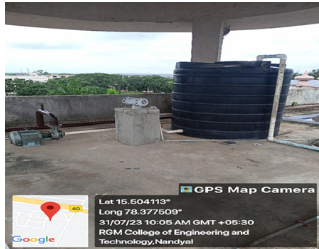
Water Tank on top of RB Block
